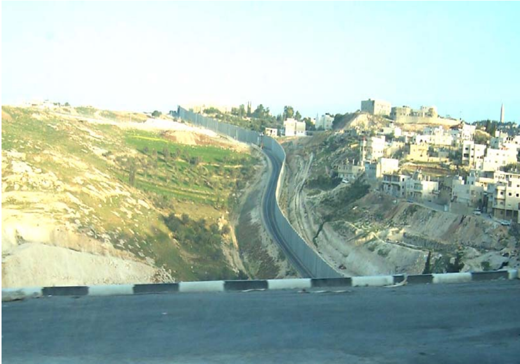
Figure 5: Section of the Separation Wall - East Jerusalem West Bank – Palestine
